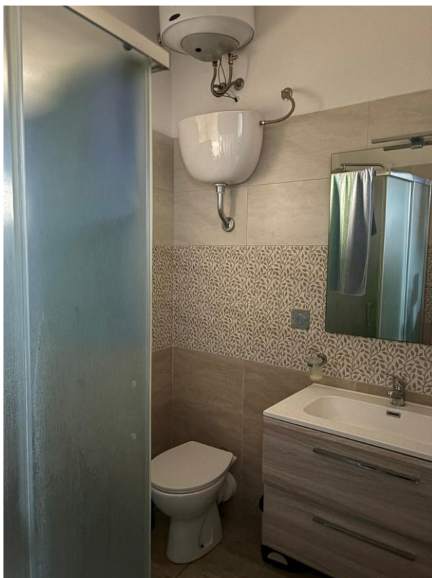
8. Piano Terra - bagno
